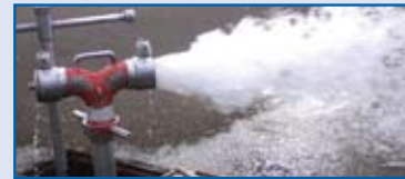
left: A fire hydrant is opened to flush out the pipes.
