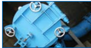
left: The swabbing chamber at Fitzherbert Bridge.
