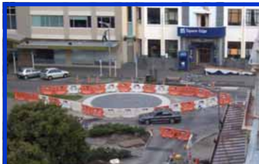
New roundabout at intersection of Church Street and The Square
