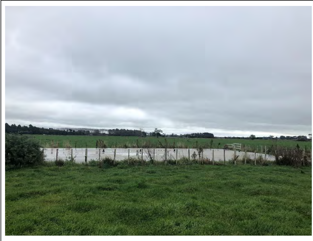
Photograph 18 Appendix B.1: Effluent pond with cover north west of the milking shed.
