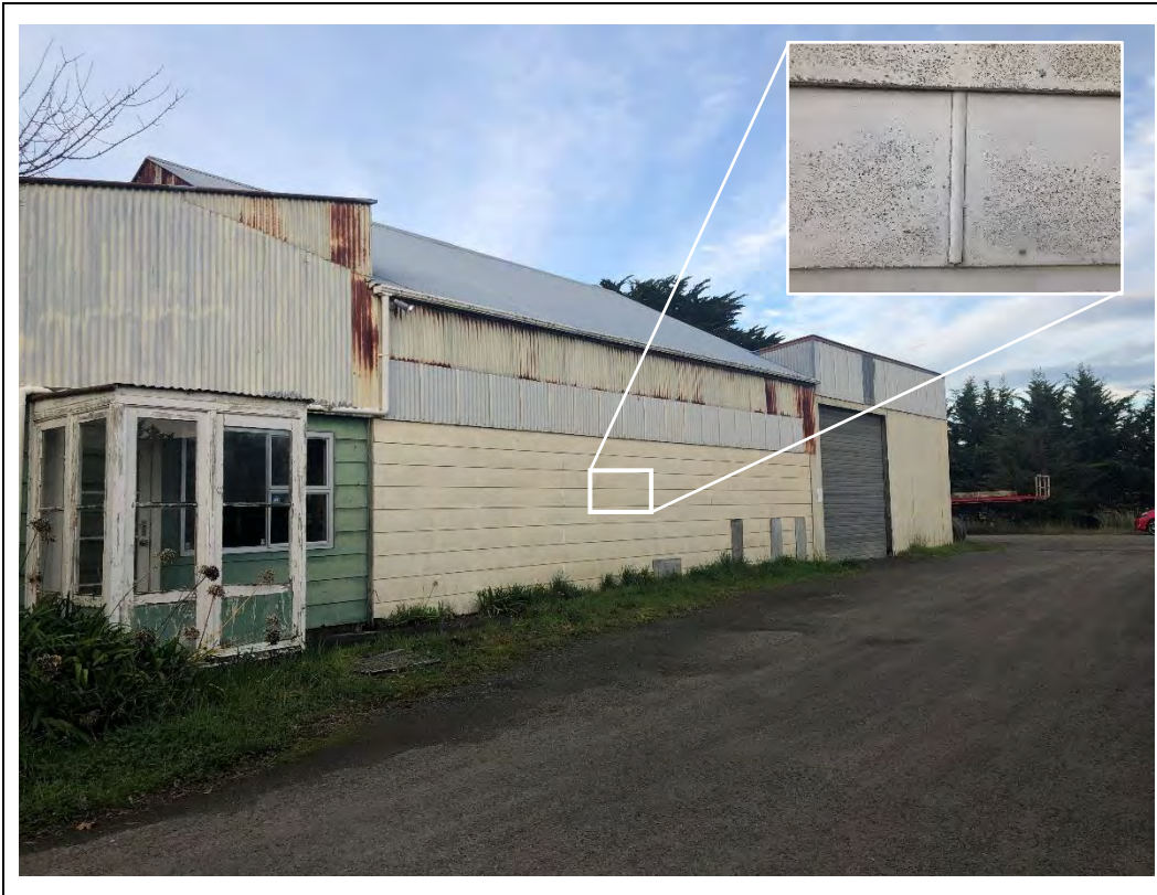
Photograph 56 Appendix B.1: Eastern portion of the workshop building showing paving and cladding.
