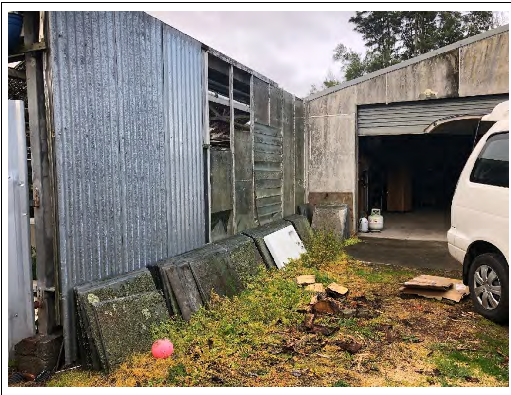
Photograph 29 Appendix B.1: Store building adjoining the southern wall of the large glasshouse.
