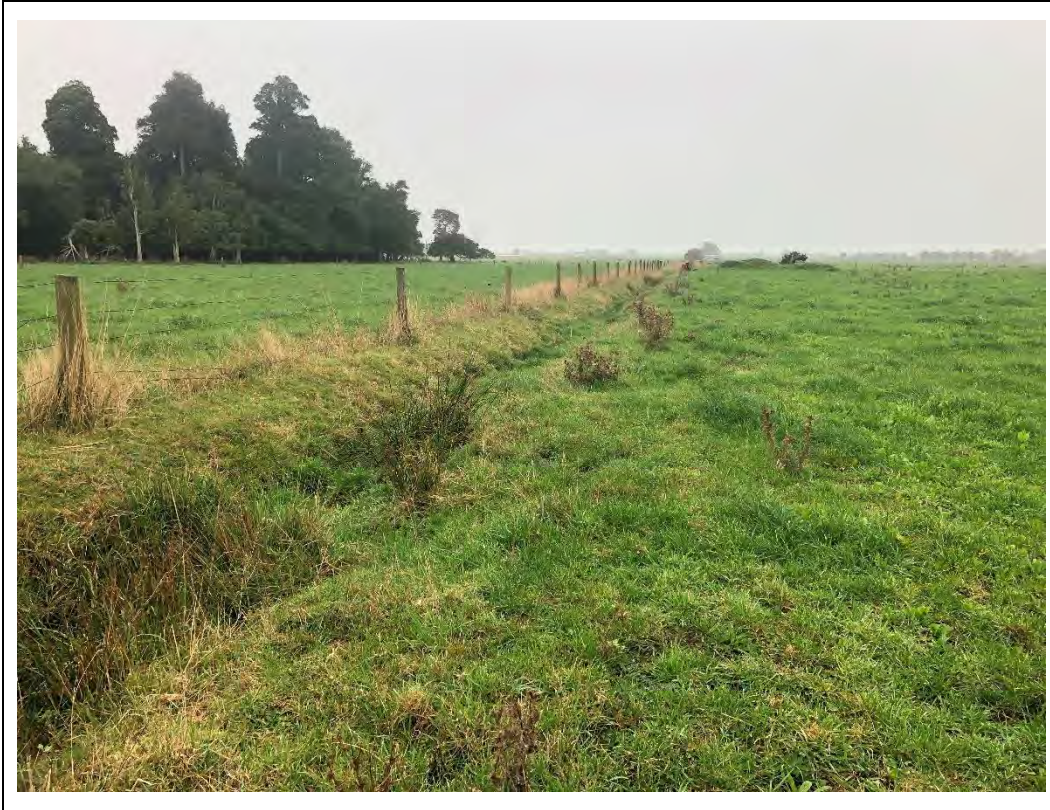
Photograph 12 Appendix B.1: Open stormwater drain extending north, dense vegetation top left of image.
