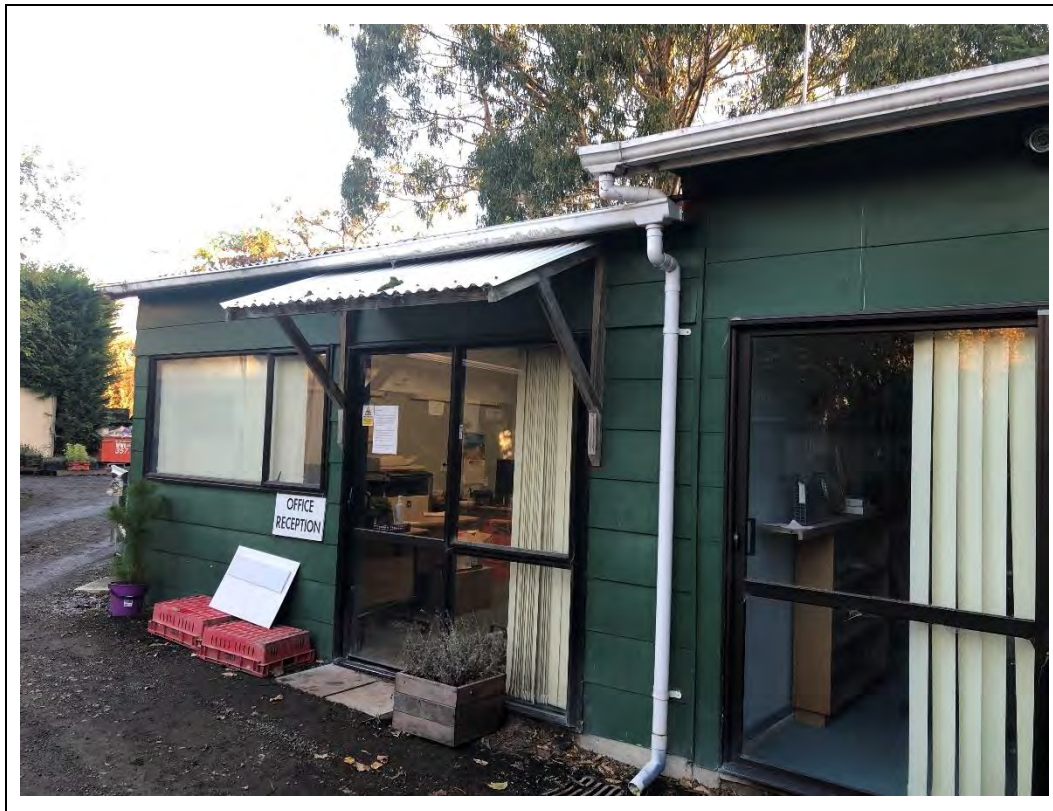
Photograph 43 Appendix B.1: Office/reception building constructed of fibreboard cladding.
