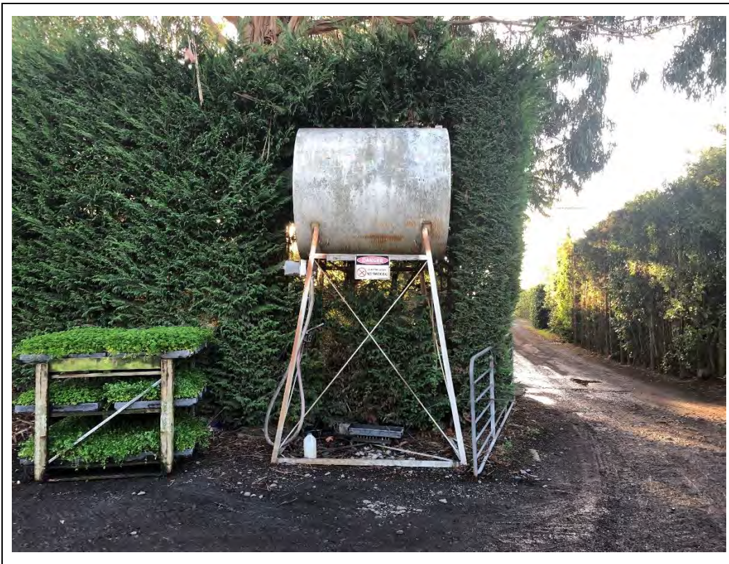
Photograph 45 Appendix B.1: Aboveground storage tank containing diesel to the west of the office building.
