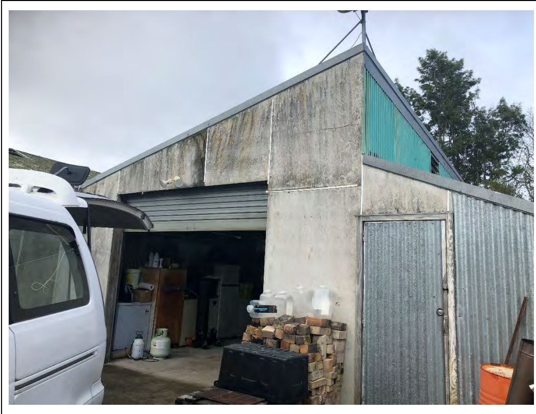
Photograph 30 Appendix B.1: Exposed fibreboard cladding on north-facing external wall of store building.
