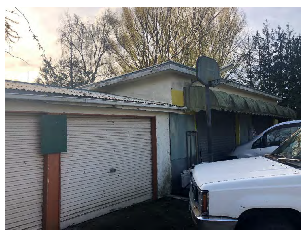
Photograph 36 Appendix B.1: Front of store/packing building constructed of fibreboard and stucco paint.
