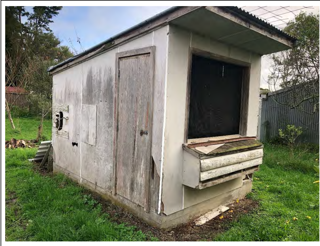
Photograph 23 Appendix B.1: Small shed constructed of fibreboard to the north of the house.
