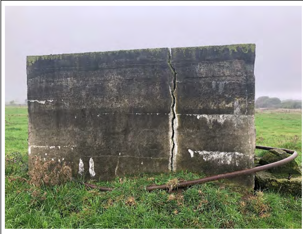
Photograph 10 Appendix B.1: Rectangular tank, pipework and cracking evident in image.
