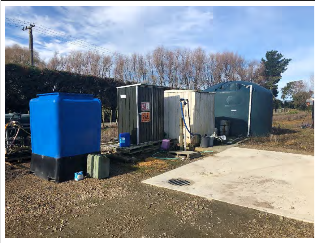
Photograph 49 Appendix B.1: Hazardous substance store, pump shed and water tank.
