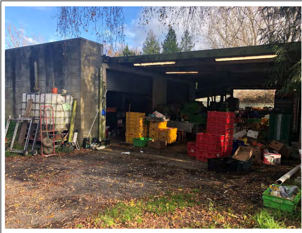
Photograph 37 Appendix B.1: Rear of store/packing building containing items including containers of oil.
