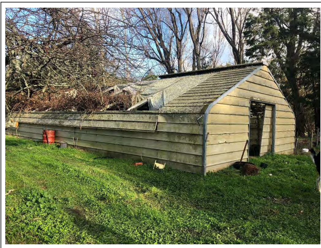
Photograph 39 Appendix B.1: Disused tunnel house to the west of the store building.
