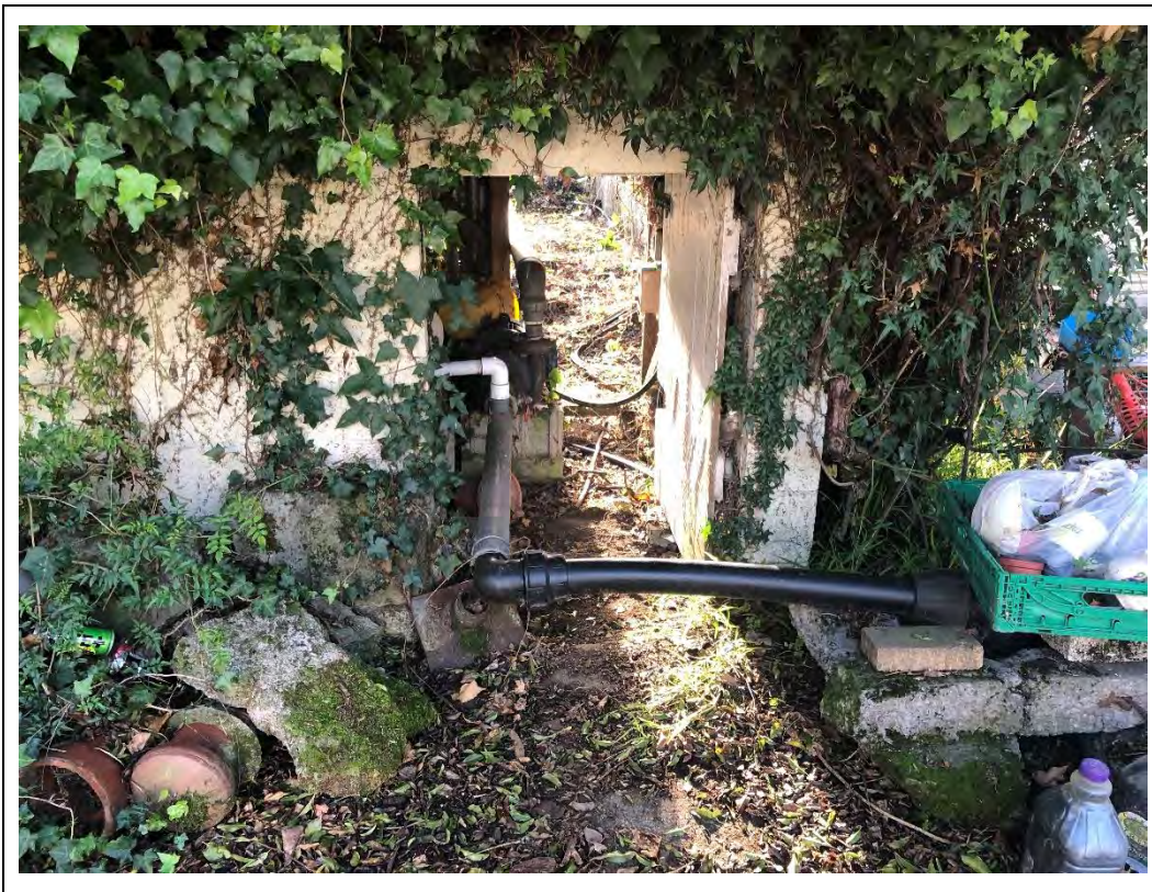
Photograph 41 Appendix B.1: Bore shed to the west of the store building, litter present at front of shed.
