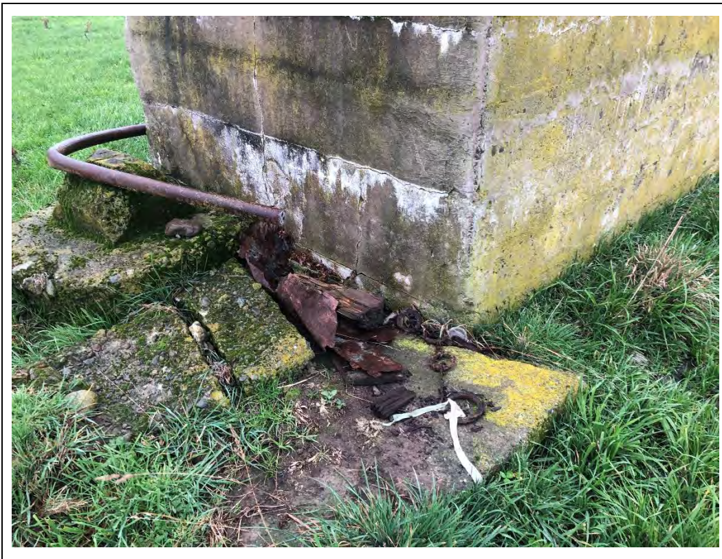
Photograph 11 Appendix B.1: Metal and concrete fragments present at base of tank.
