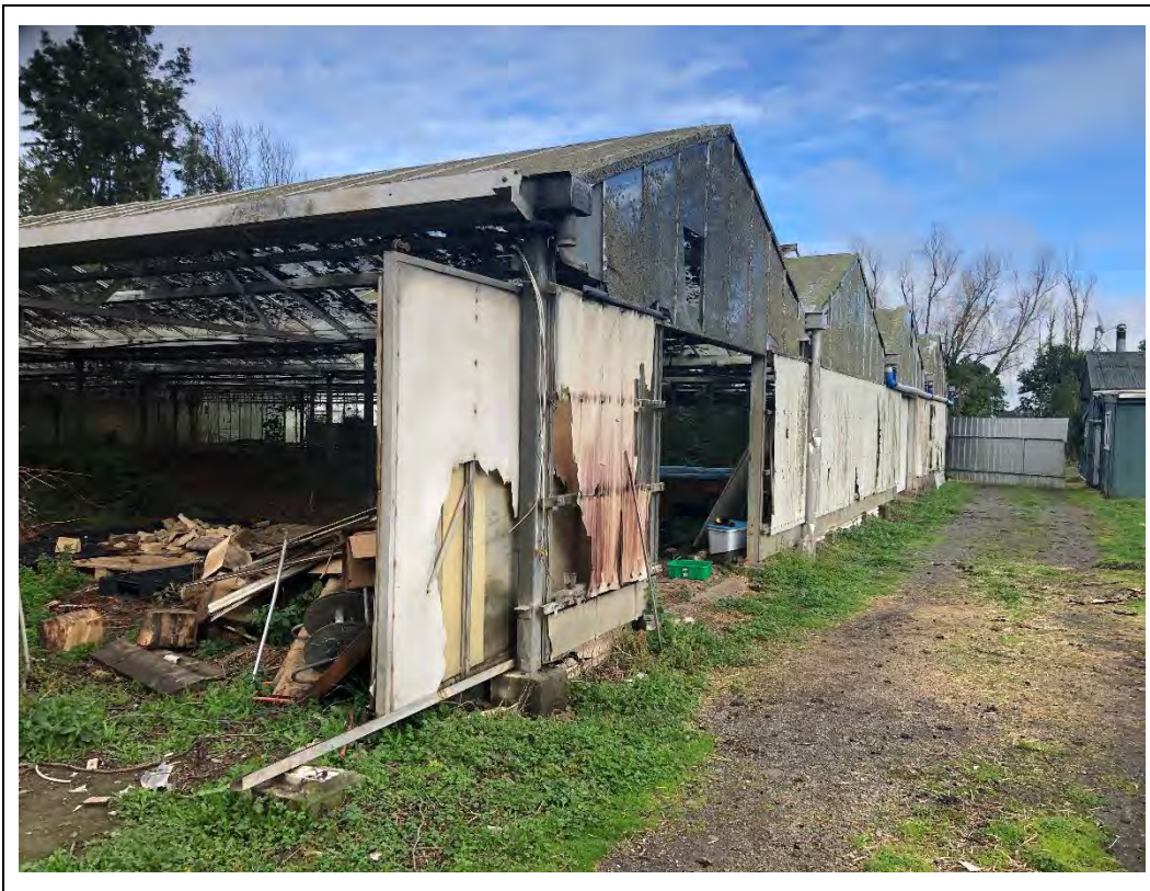
Photograph 31 Appendix B.1: Southern portion of disused and deteriorating commercial glasshouses.
