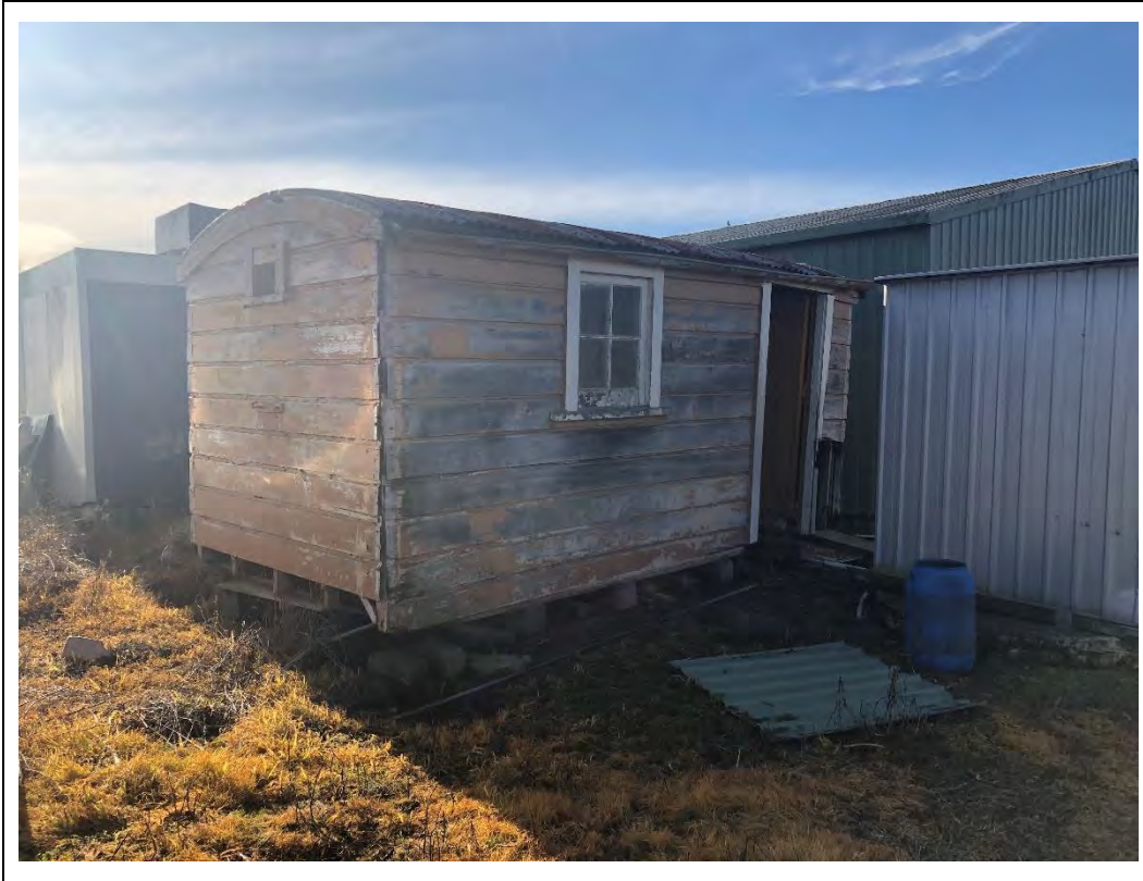
Photograph 51 Appendix B.1: Small timber building with flaking paint to the west of the main building.
