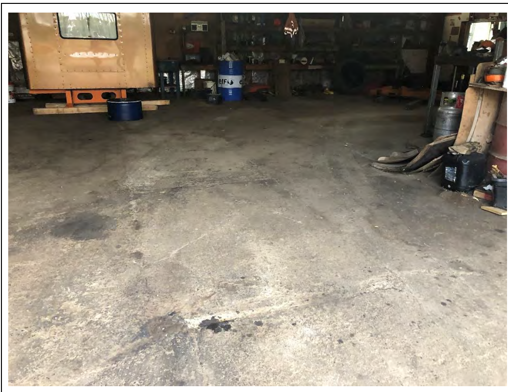
Photograph 57 Appendix B.1: Within workshop building looking towards shelving on eastern wall. Cut rectangular area within concrete floor. Hydrocarbon staining evident.
