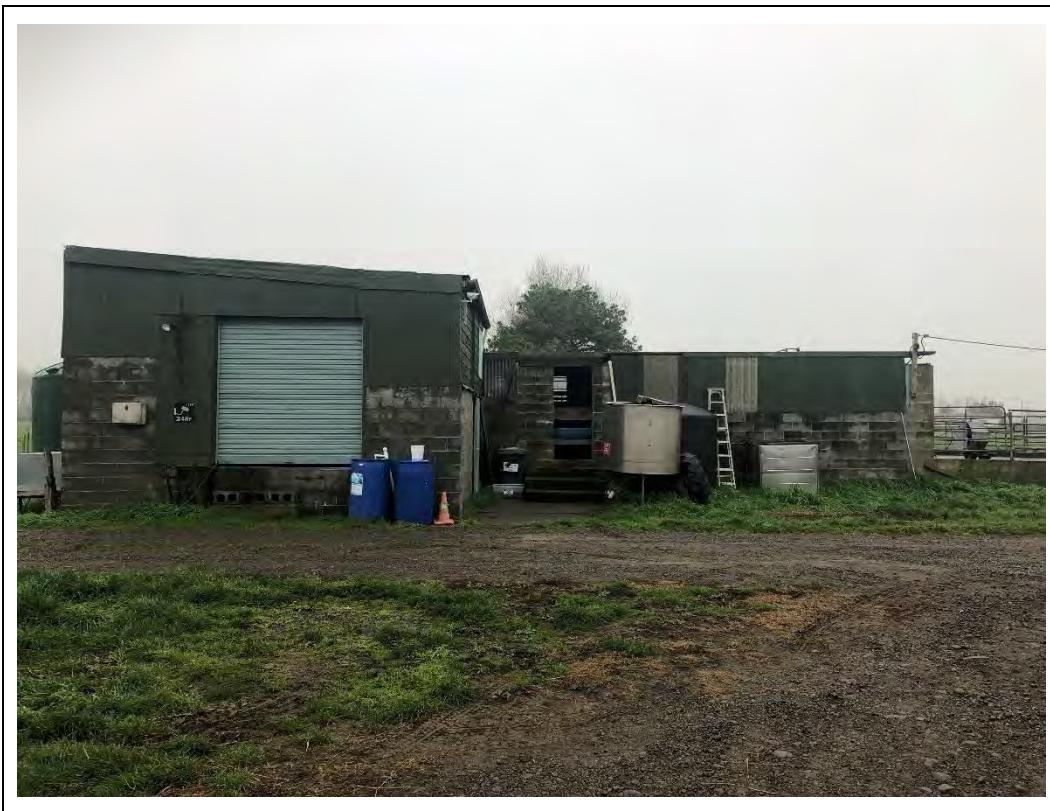
Photograph 2 Appendix B.1: Milking shed constructed of cinderblock, corrugated iron and 'clearlite' panels.
