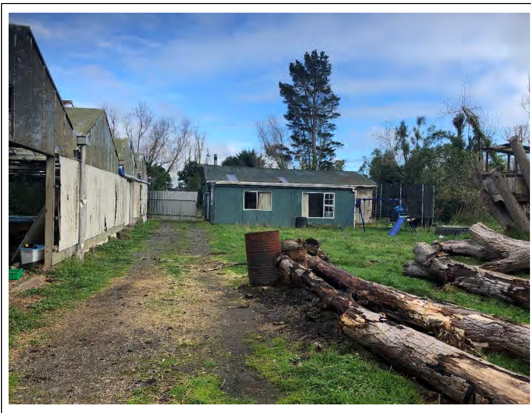
Photograph 27 Appendix B.1: Rear of office/retail building showing board and batten style cladding.
