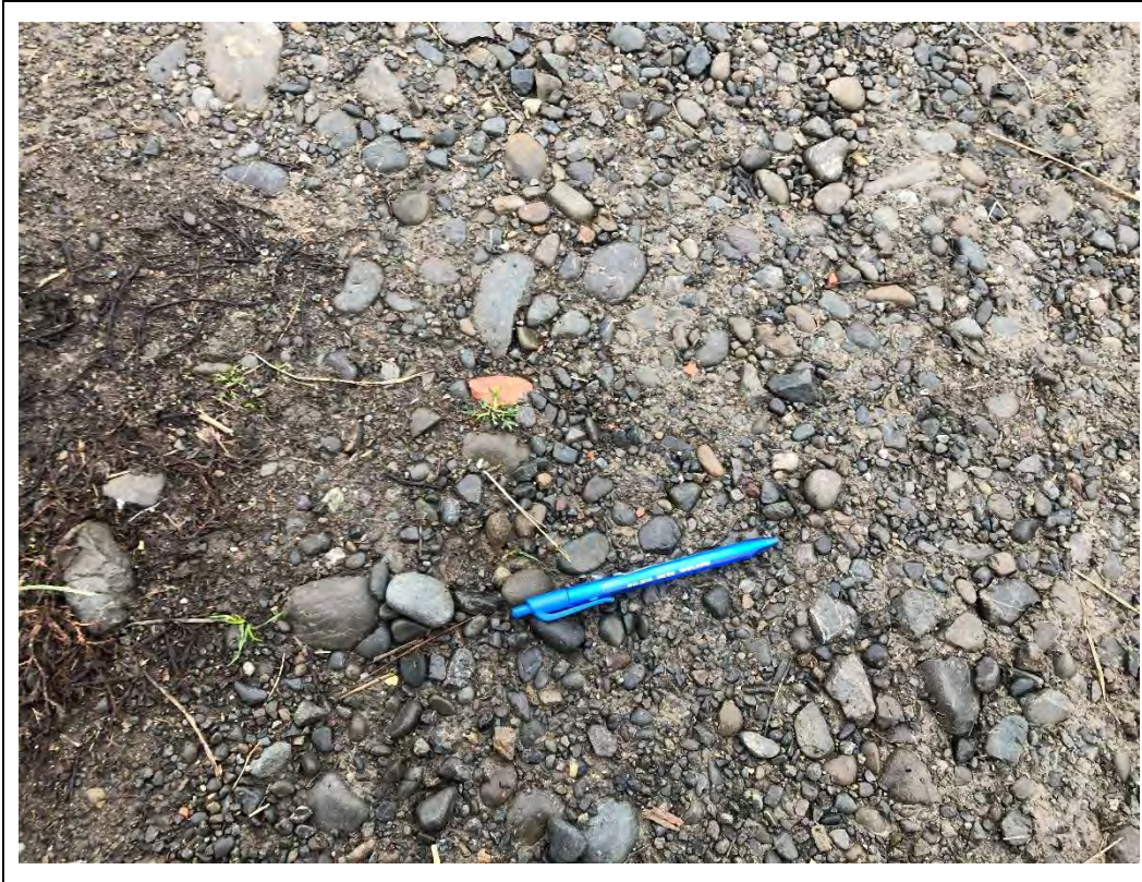
Photograph 3 Appendix B.1: Brick fragments observed in driveway.
