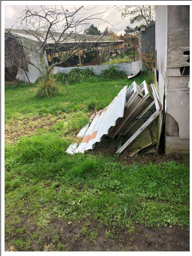
Photograph 25 Appendix B.1: Building material stored to the rear of the small shed.
