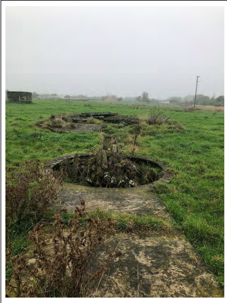
Photograph 9 Appendix B.1: Remnants of former plunge sheep dip filled with concrete and fenceposts to prevent stock access, looking north east. Rectangular tank visible beyond the dip.
