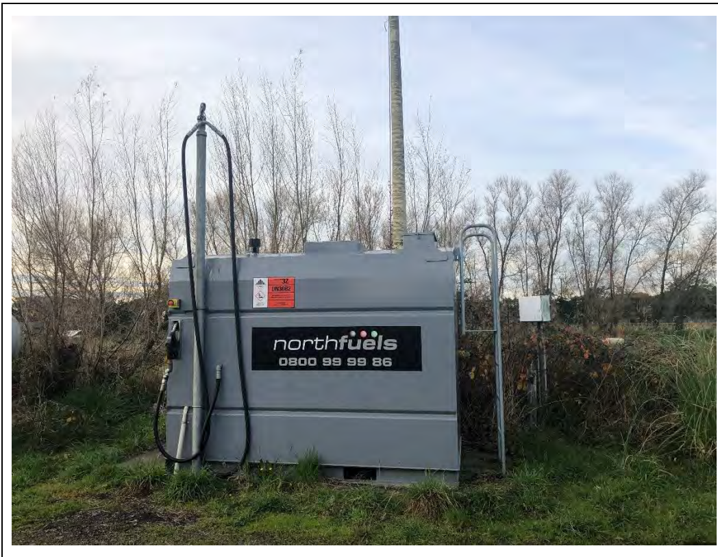
Photograph 59 Appendix B.1: Aboveground storage tank on western portion of the property.
