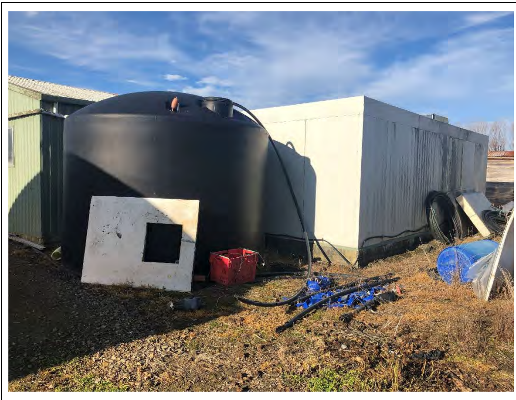
Photograph 52 Appendix B.1: Water tank and refrigerated building to the west of the main building.
