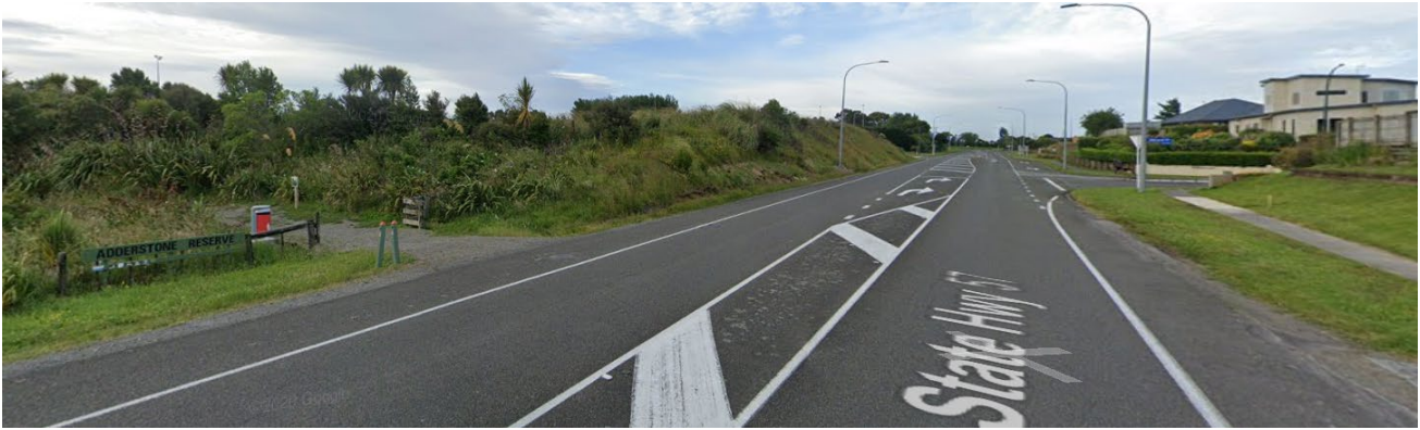
Figure 12: Pedestrian Access to the Adderstone Reserve from SH57 (extract from Google Streetview)
