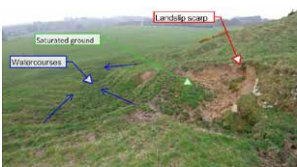
Photograph 10: Voss block: water induced landslips and watercourses
