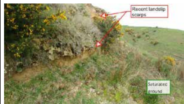
Photograph 9b: Voss block; recent landslips and saturated ground
