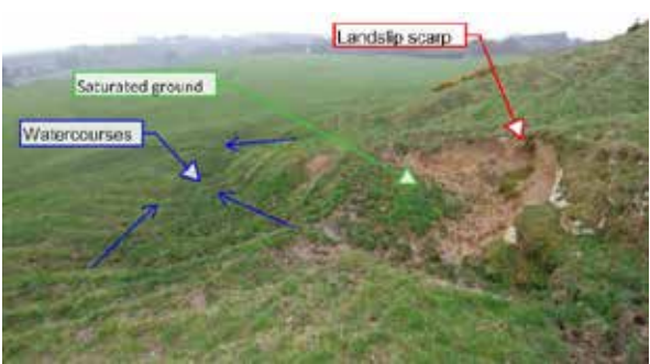
Photograph 10: Voss block: water induced landslips and watercourses
