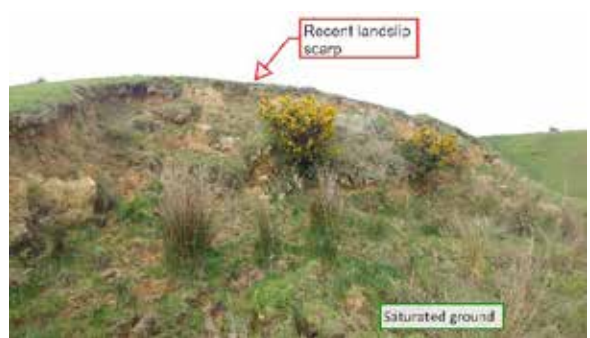
Photograph 9: Voss block; recent landslip scarp and saturated ground
