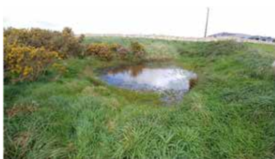
Photograph 6: Les Fugle block, standing water created by fill dam.
