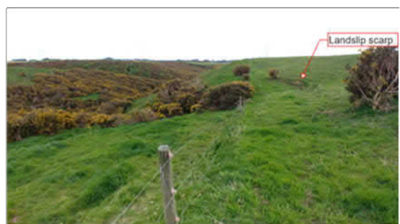
Photograph 7: Green block; historic landslip scarp
