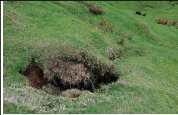
Photograph 21: Waters block; Tunnel gully erosion
