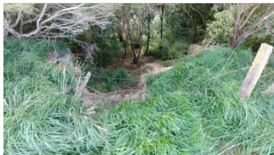
Photograph 4: Les Fugle block; recent landslip
