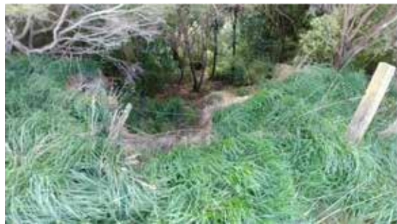
Photograph 4: Les Fugle block; recent landslip
