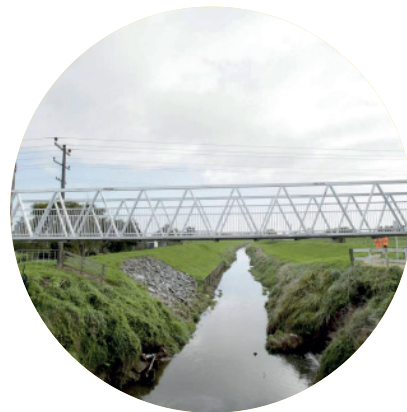
Bridge over the channelised stream
