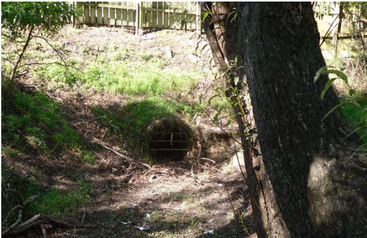
Figure 9: PNCC Stormwater Connection adjacent to 91 Benmore Avenue.
