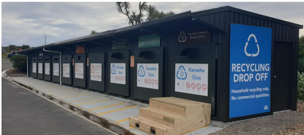
Figure 32: The New Awapuni RDOP
