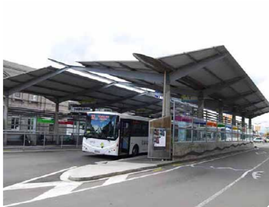
Image 70: Main Street Urban Bus Terminal
