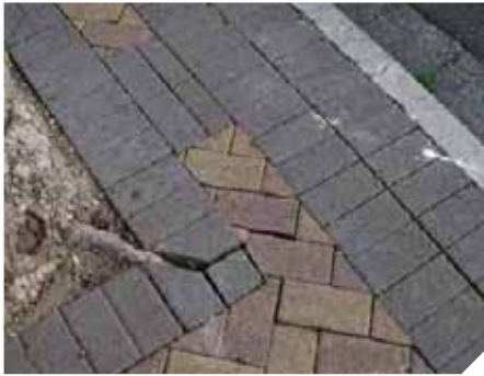
Image 81: Clay paving / tree pit detail
