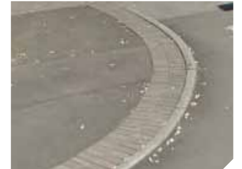
Image 89: Concrete kerbs with clay paver
