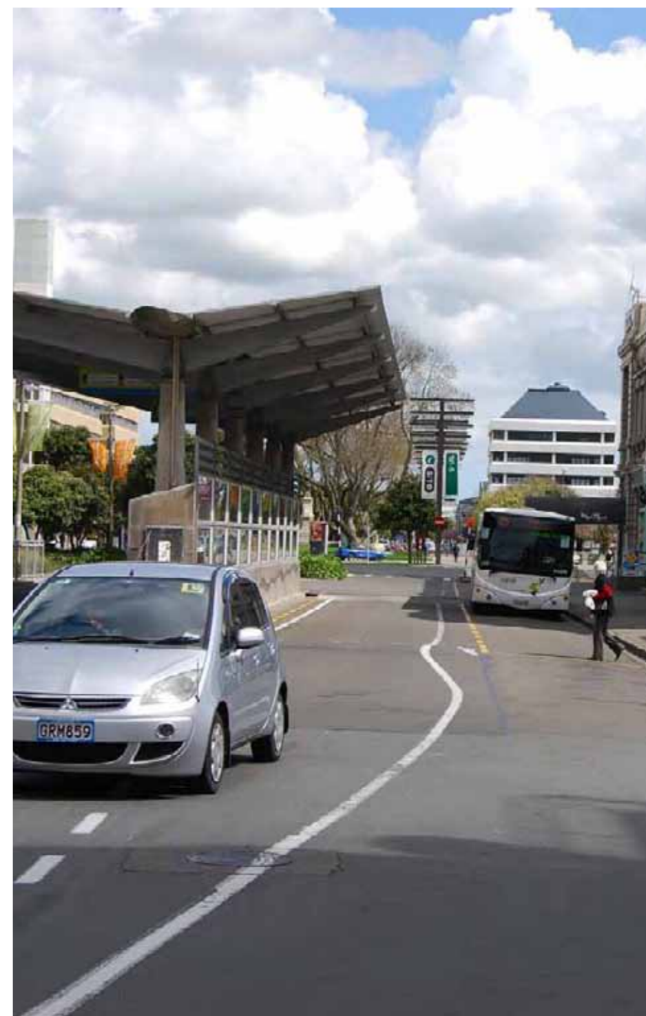
Image 5: Main Street - Urban Bus Terminal
