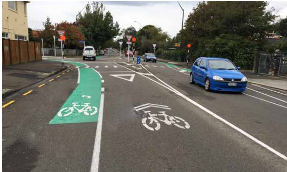
Figure 16: Cycle lanes up to and through a roundabout only work on three-leg roundabouts (Featherston Street/Freyberg Street)
