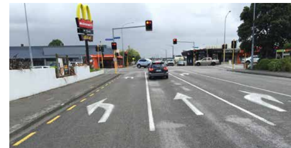
Figure 10: Existing conditions on Featherston Street at Rangitikei Street
