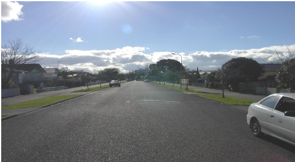
Residential Street before treatment
