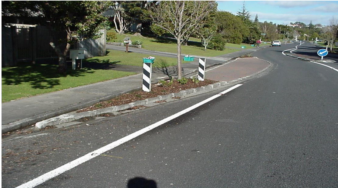
Photograph 5 - Chicane with two way flow
