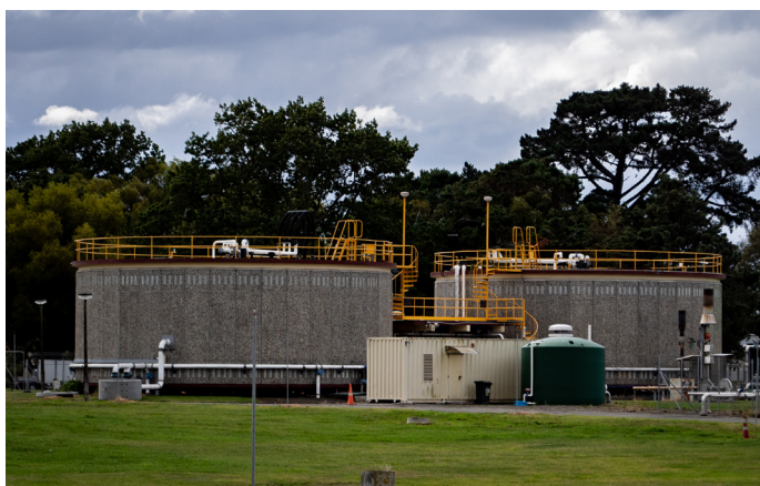
Solid material removed from wastewater is broken down by bacteria in these tanks for 20 days and is then taken off site.
