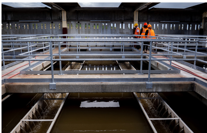
Water is held in these tanks where solid material sinks and clean water flows on to the next stage of treatment
