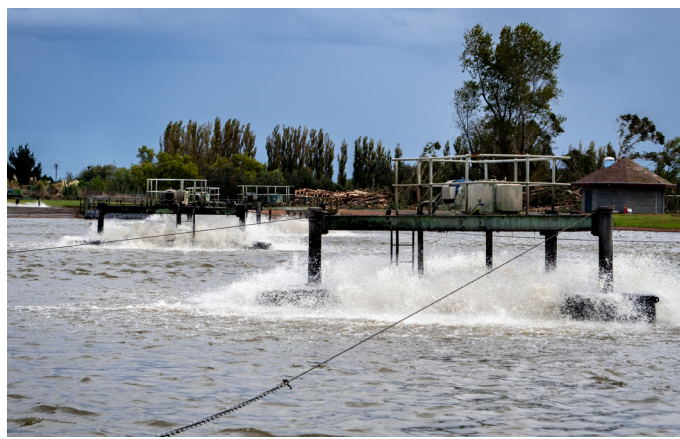
Air is pumped into water to provide oxygen to microorganisms that consume any remaining solid material in the wastewater.
