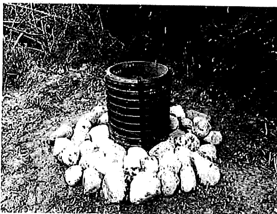
Figure 1: Example of a manhole type energy dissipating structure
