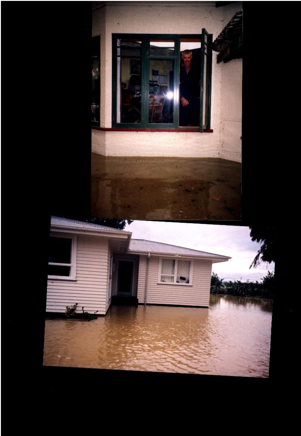
Mangaone Stream Floods 2004 Flyers Line
