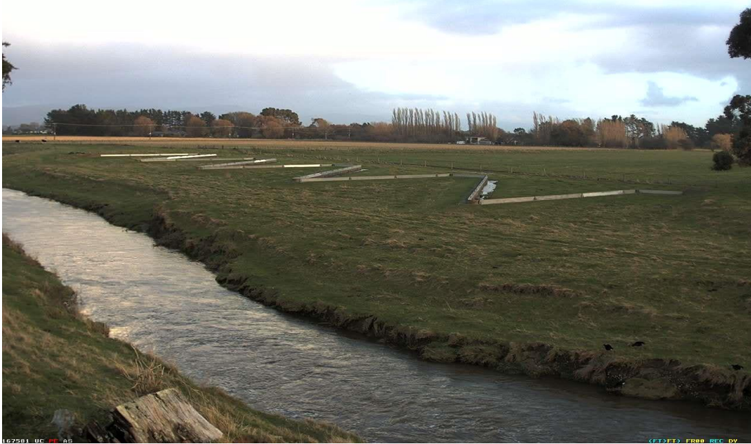
Flyers Line Spillway (no allowance flooding that occurs above spillway 2/6/22)
