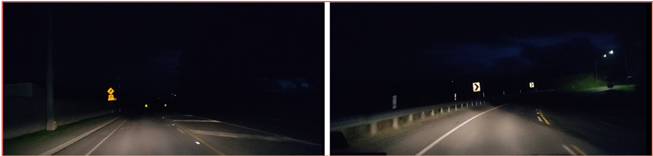
Figure 29: Inconsistent lighting in miblock between Johnstone Drive and Cashmere Drive
