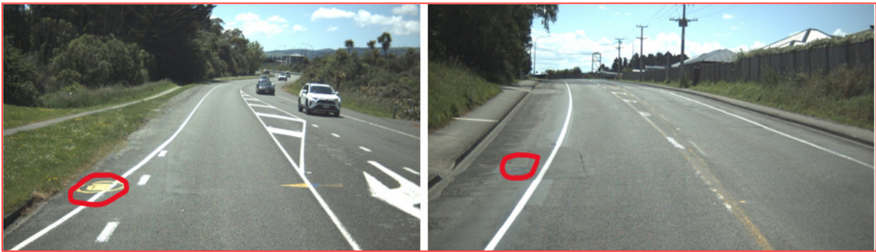
Figure 43: Service covers along Northbound of Aokautere Drive
