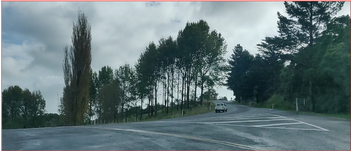
Figure 18: Superelevation at Turitea Road/ SH57 Old West Road Intersection
