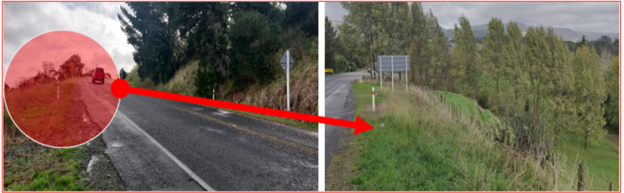
Figure 33: Drop-off on SH57 Old West Road - Northbound
