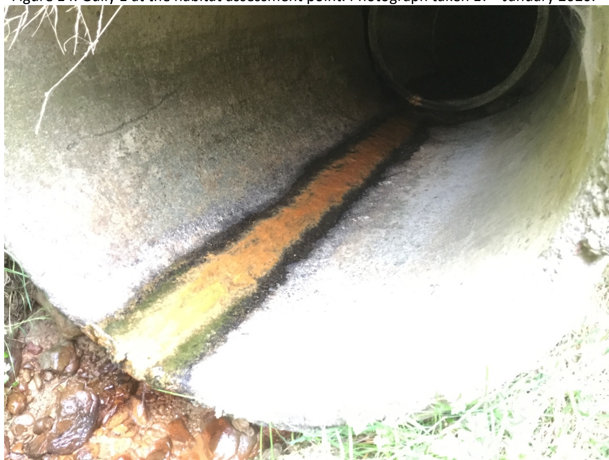
Figure 15. Gully 3 showing the perched culvert (with perched culvert extension) at the location shown in Figure 1. Photograph taken 17 th January 2020.
