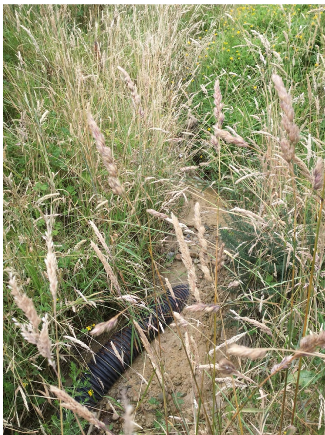
Figure 10. Gully 1 within 10 m downstream of the c.3-4 m tall cliff, which is at the transition point between permanent and intermittent stream hydrosystems (point A, Figure 1). The photograph shows permeable piping embedded in the stream bed presumably acting as a discharge point from the upstream area. Photograph taken 17 th January 2020.
