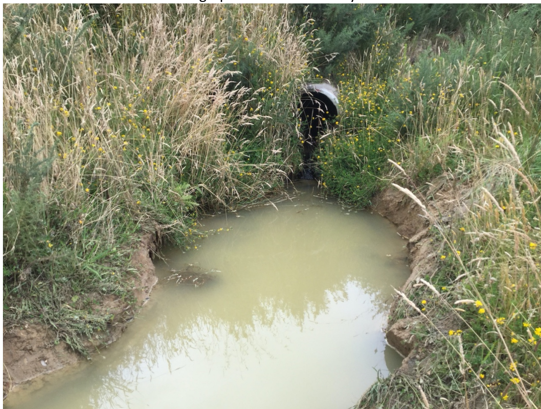
Figure 13. Gully 1 showing perched culvert at the location marked on Figure 1. Photograph taken 17 th January 2020.
