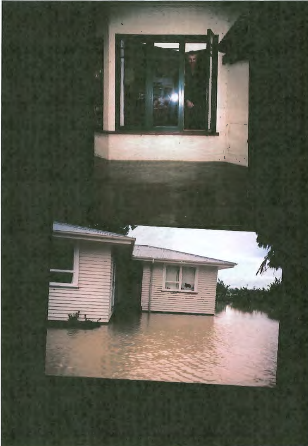
Mangaone Stream Floods 2004 Flyers Line
