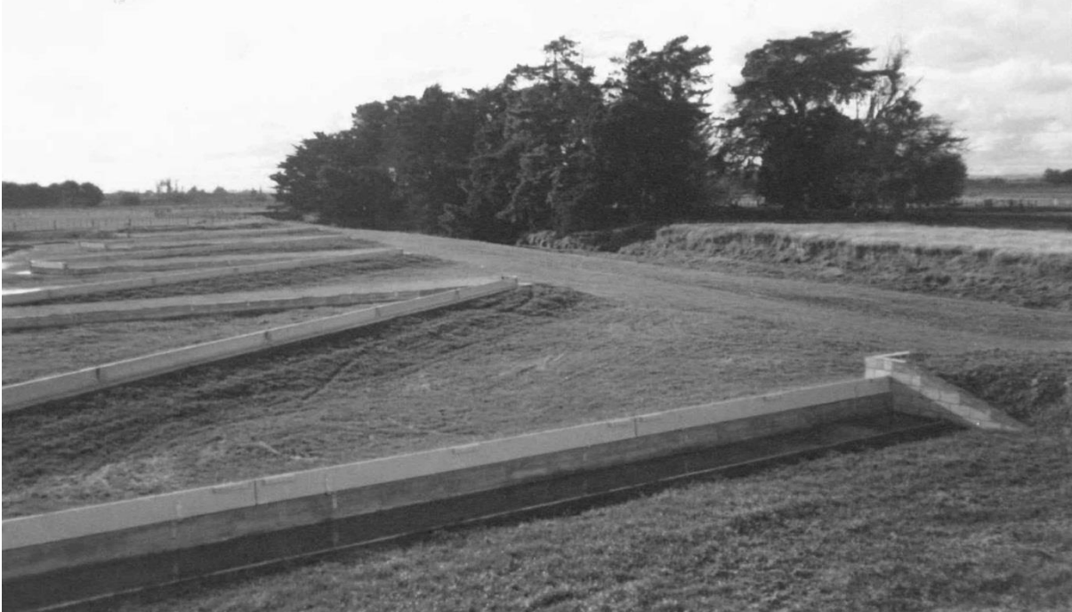
Figure 10.3.1 Flyers Line spillway from downstream end
