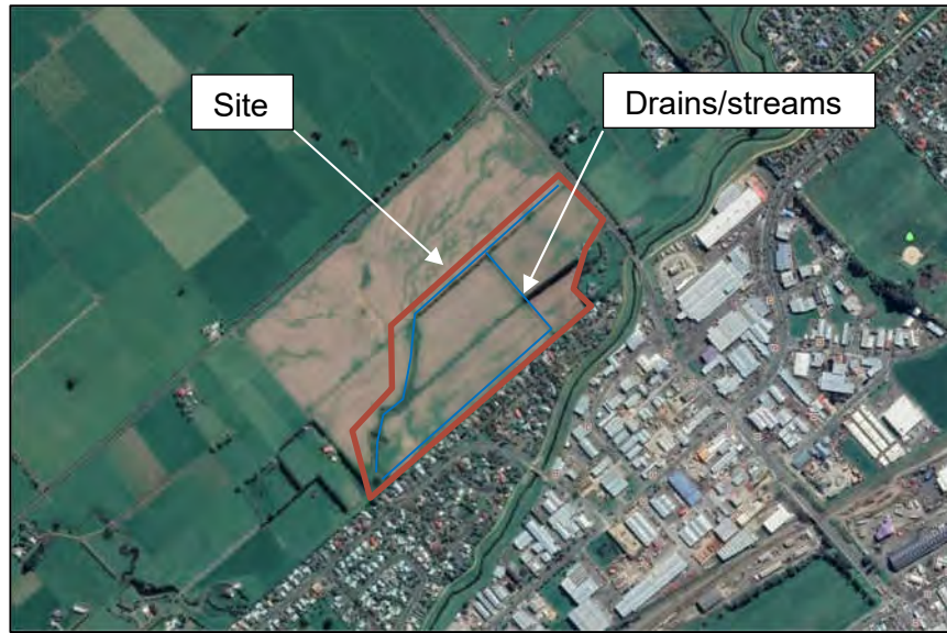
Figure 2, Google Earth image showing approximate extend of development and drainage systems
