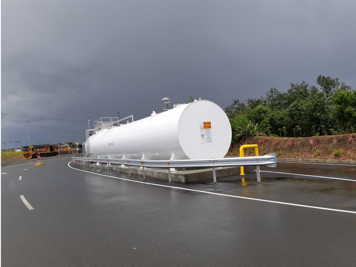
Figure 1-1 100,000l diesel tank at Westfield railway
