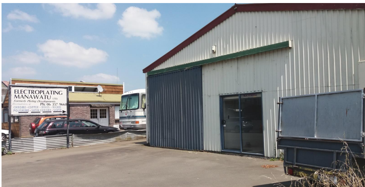
Photograph 13b: 17 Roxburgh Crescent – Asbestos cement on exterior of a building on site identified in Property files held by PNCC
