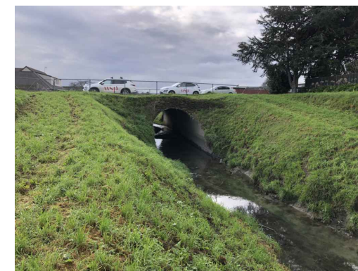
IMAGE - CULVERT OUTLET
