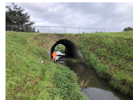
IMAGE - CULVERT INLET
