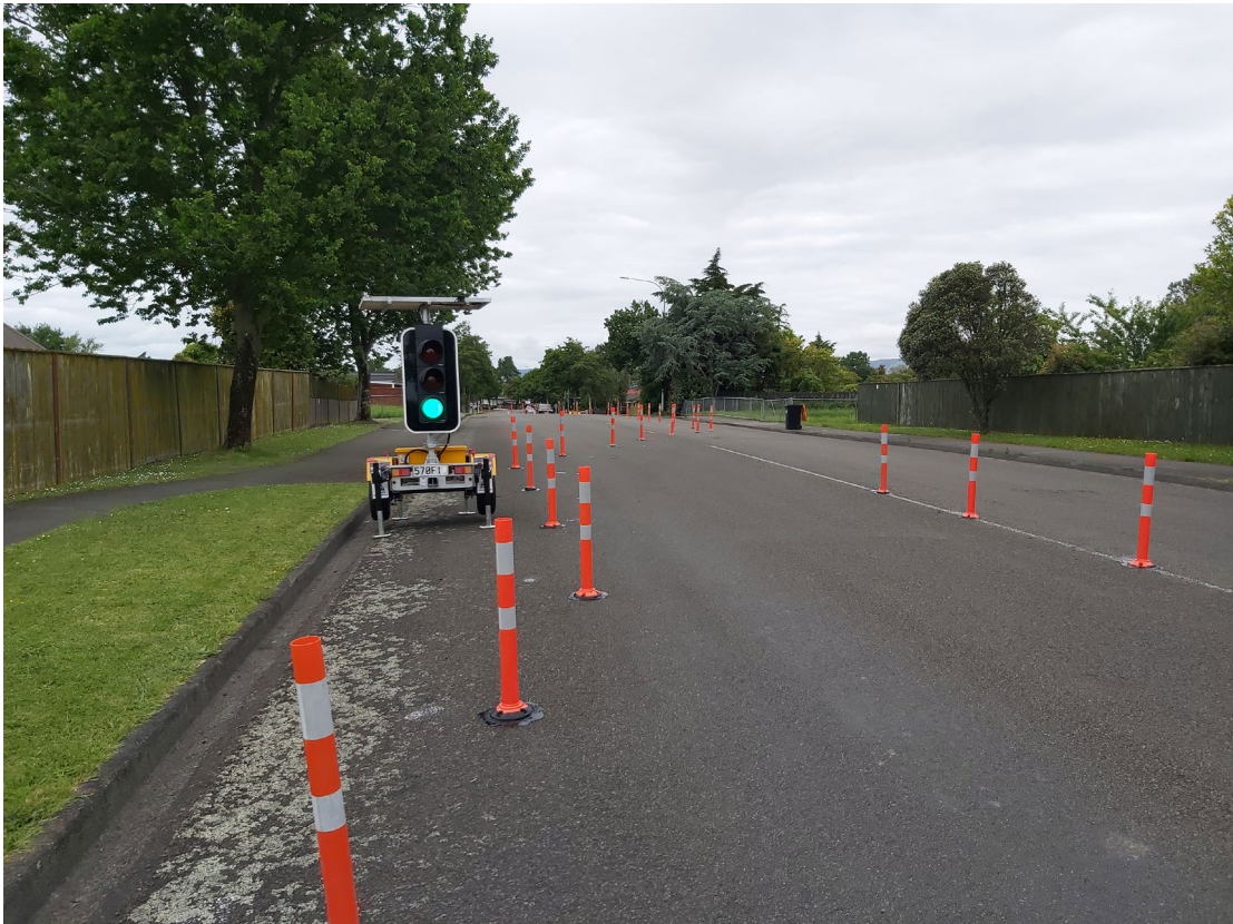
Figure 3 photo: traffic management in place on Amberley Ave.
