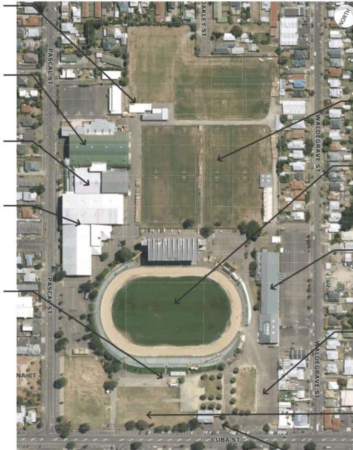
CETA key facilities
