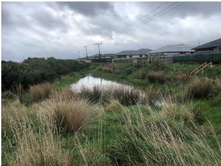
Figure 6: Bunded Stormwater Discharge From Monaco Grove.
