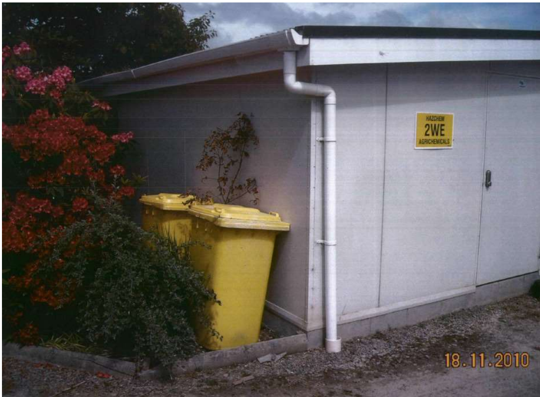
Figure 4 - Photo of chemical storage shed with HazChem signage
