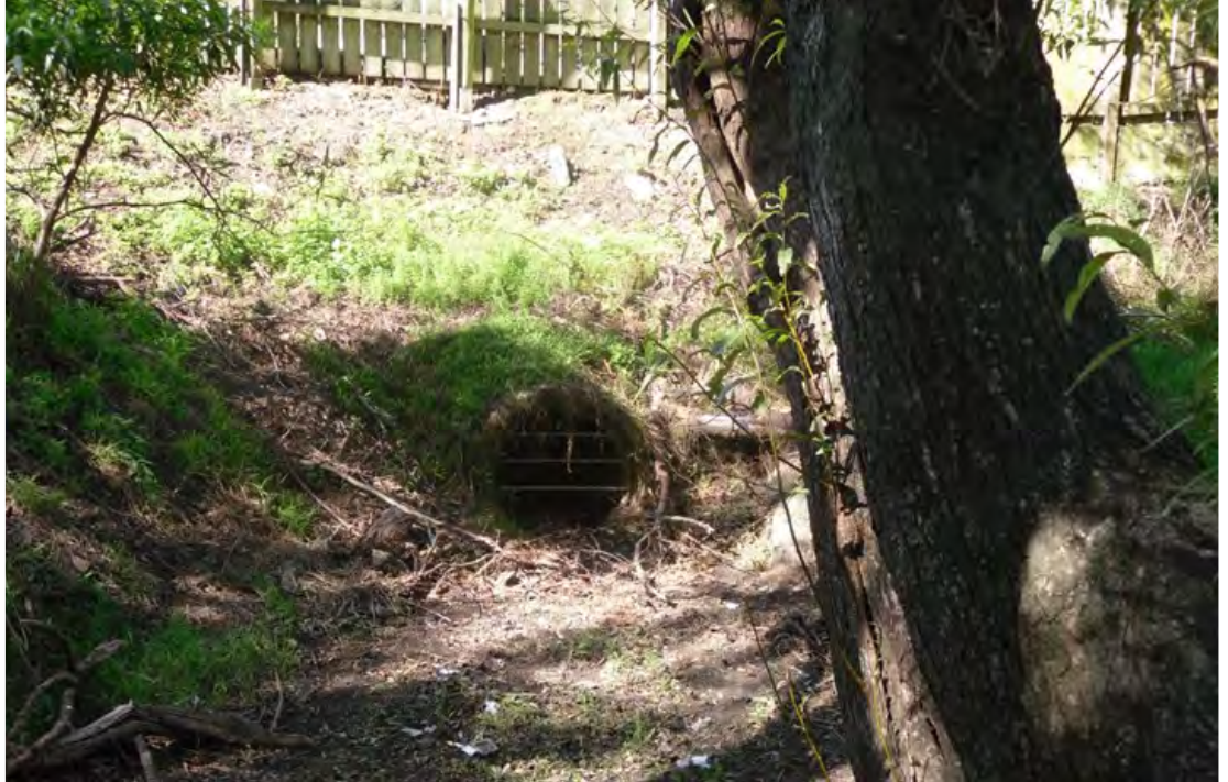
Figure 1: PNCC 900mm dia. stormwater connection at 91 Benmore Avenue
