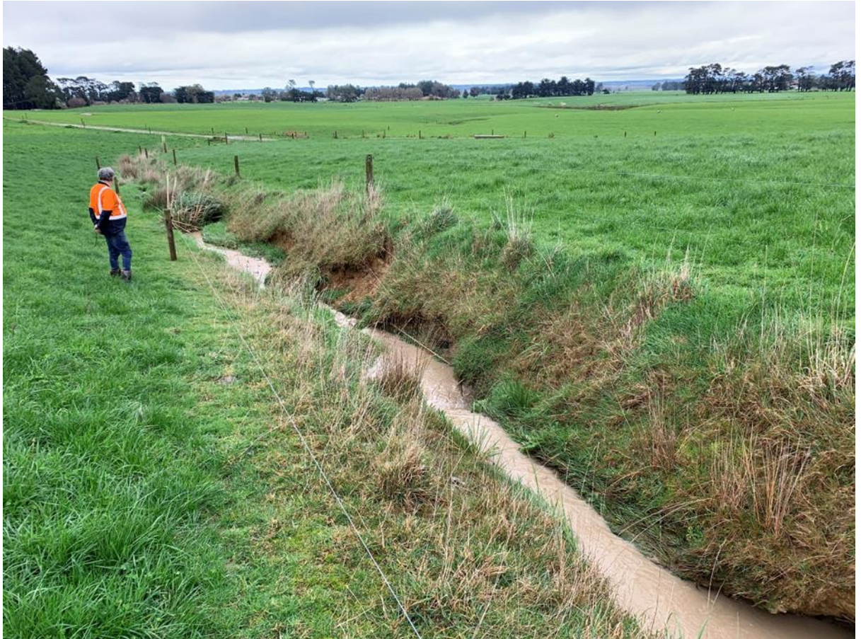
Figure 6: The unnamed tributary (Farm drain) from the same spot as Figure 3 looking downstream towards the farm. It has a clearly defined channel and visual inspection determined that the colour/clarity of the water was poor.
