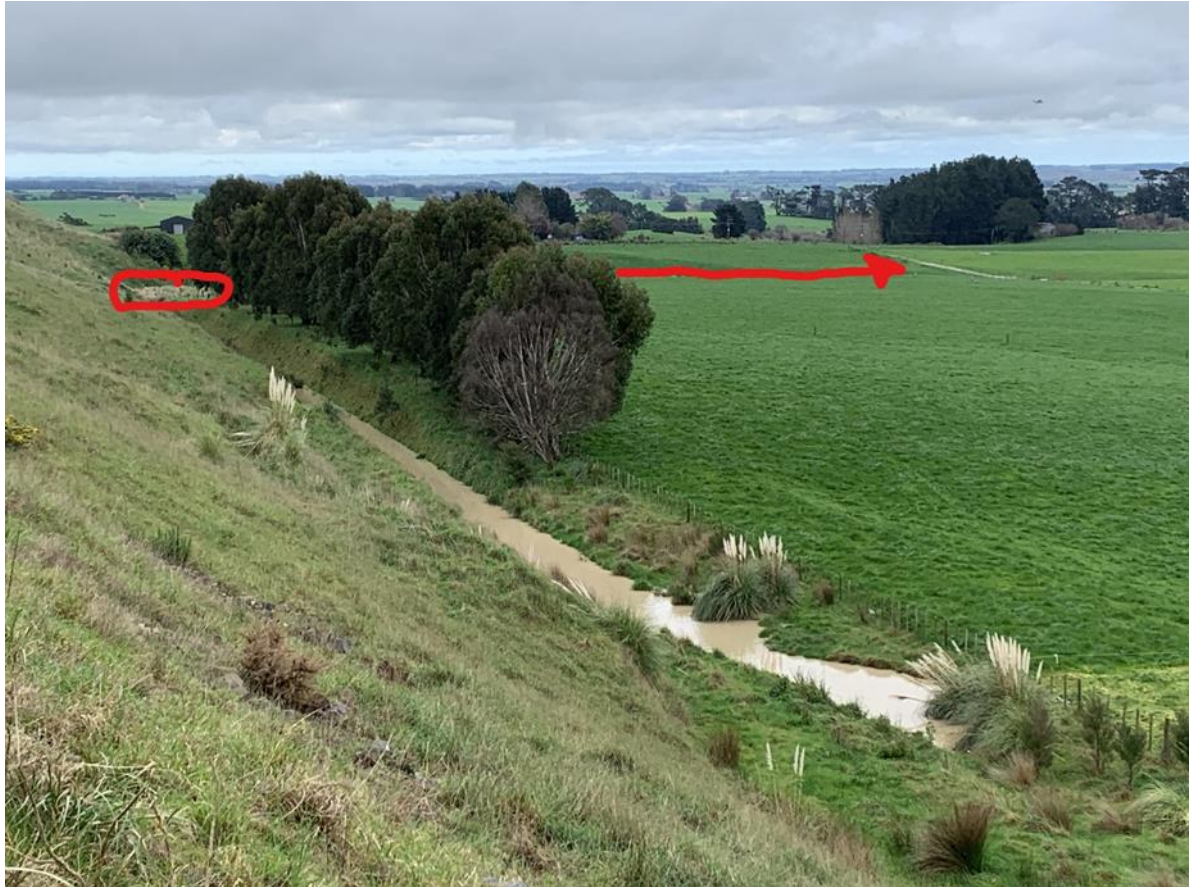
Figure 2: This image shows the ponding area parallel to the bund. The assumption is that the pooled area is an accumulation of the storm water discharging off site through the three discharge points along the bund. The red arrow shows where the farm drain referred to in the application is flowing and the red circled area is the Raupō dominated area at the top of the Farm drain.
