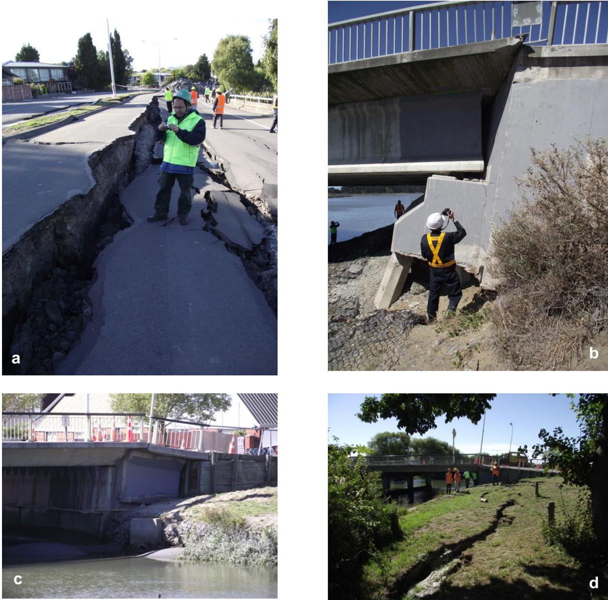
Figure 2 These photos provide examples of lateral spreading and settlement adjacent to the Avon River after the Christchurch Earthquake: a) Fitzherbert Terrace near the junction with Avonside Drive; b) Bridge St. bridge near New Brighton showing abutment settlement and rotation; c) the Avondale Rd. bridge with lateral spreading cracks and d) abutment rotation and settlement.
