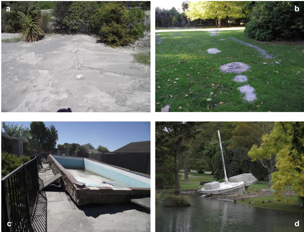
Figure 1 Photos from Christchurch showing evidence of liquefaction in the form of sand boils along “fissures”. a) The Avon River right bank at Anzac Bridge. b) Mona Vale gardens in Fendalton. c) This swimming pool was full of water during the Darfield Earthquake and stayed in the ground when the site liquefied. However, it was empty and “floated” when the site liquefied in the Christchurch Earthquake. d) This pumping station caisson floated and moved laterally during both earthquakes.
