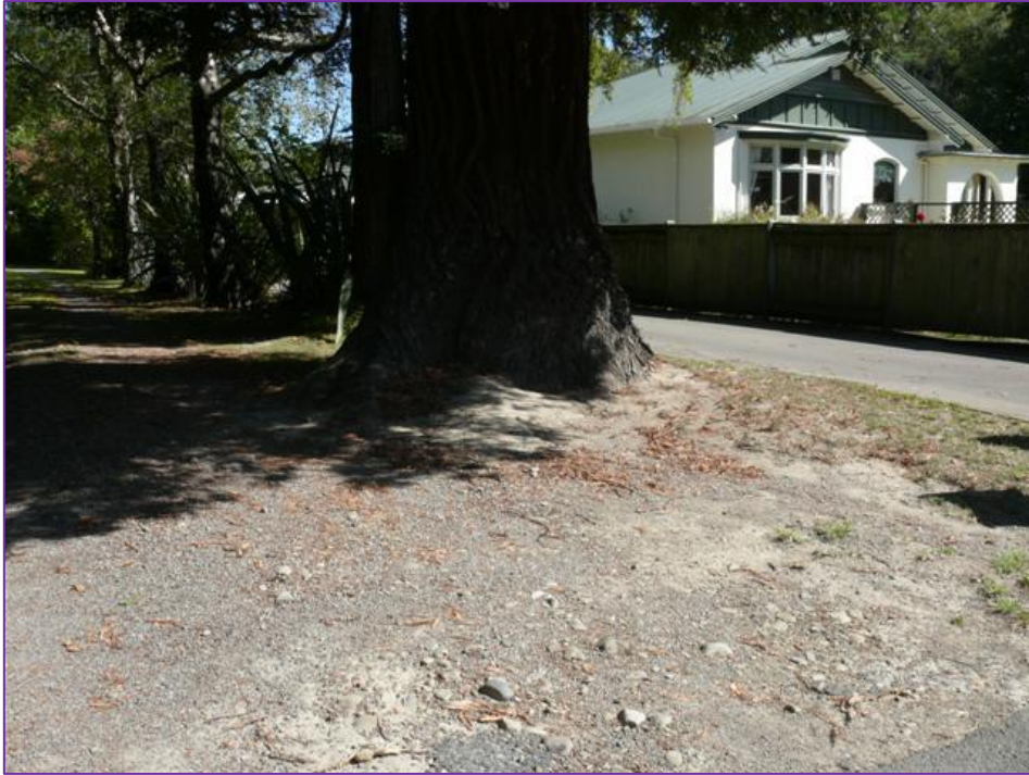
Figure 2. Base of tree, showing the limited grow space available for the root system.
