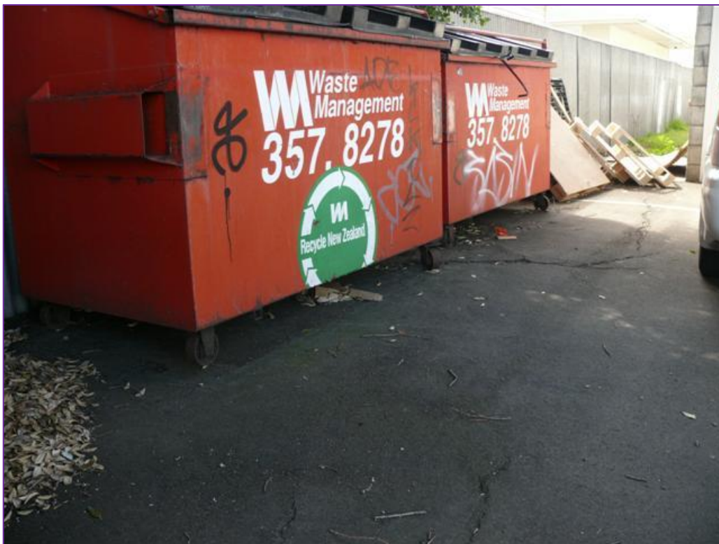
Figure 3. cracks appearing in the car park surface.
