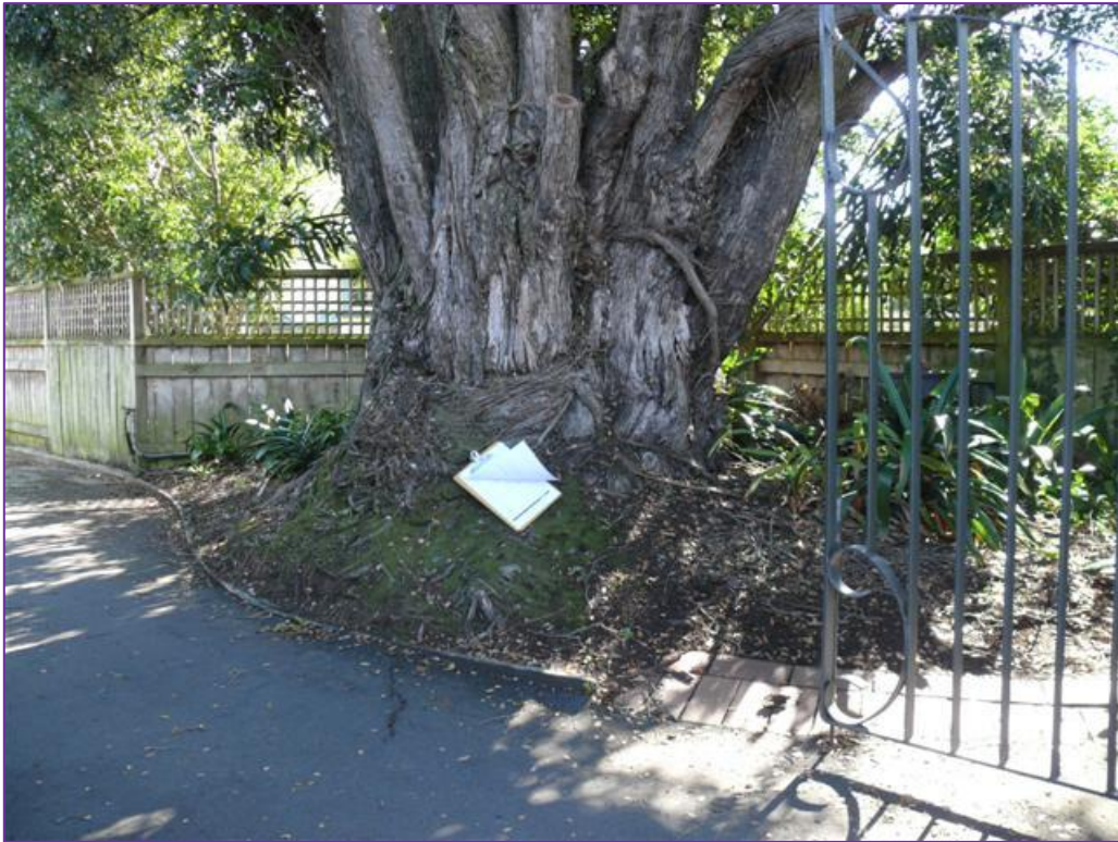
Figure 6. The tree has survived a considerable amount of root pruning. The driveway will continue to crack and should be repaired frequently
