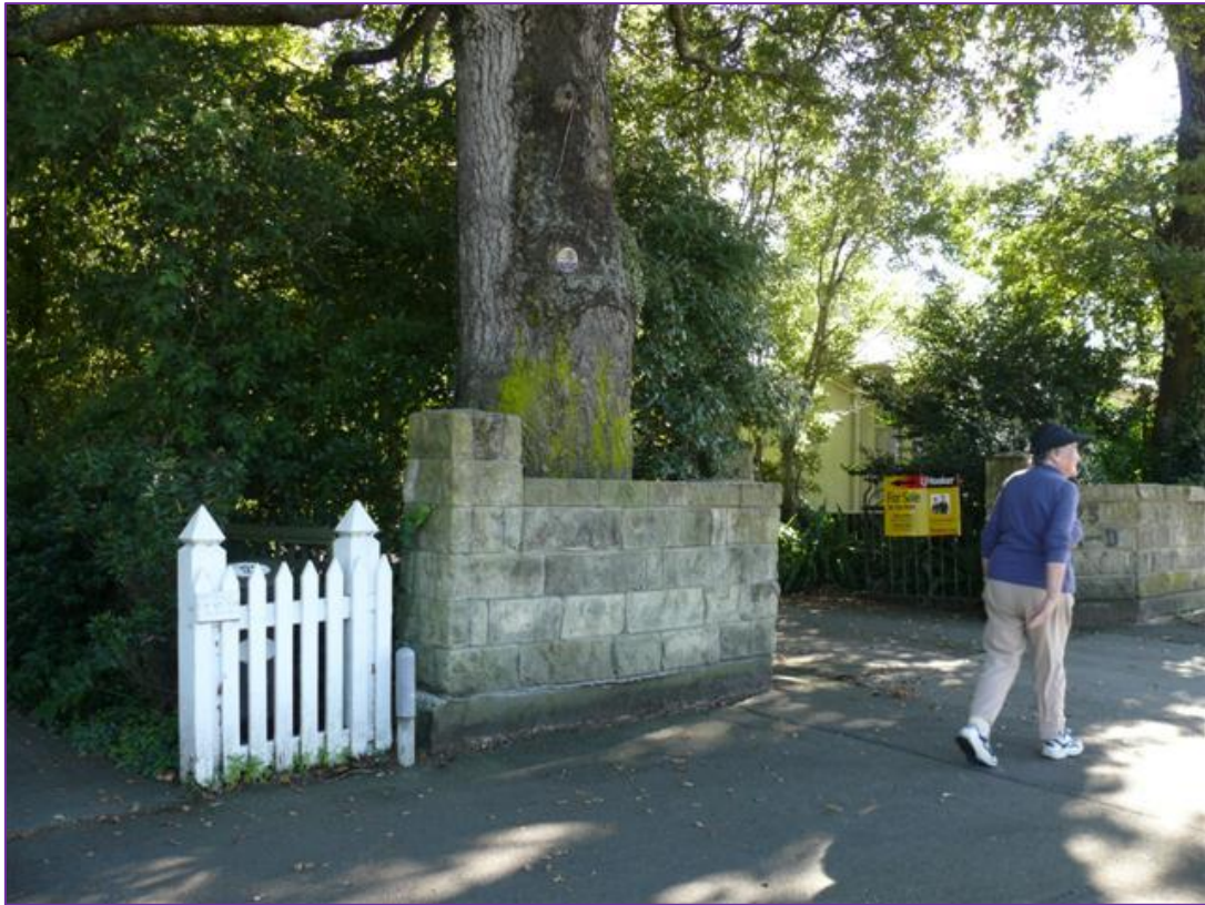
Figure 3, the tree in its setting – note the newly patched asphalt where a trench had been dug.
