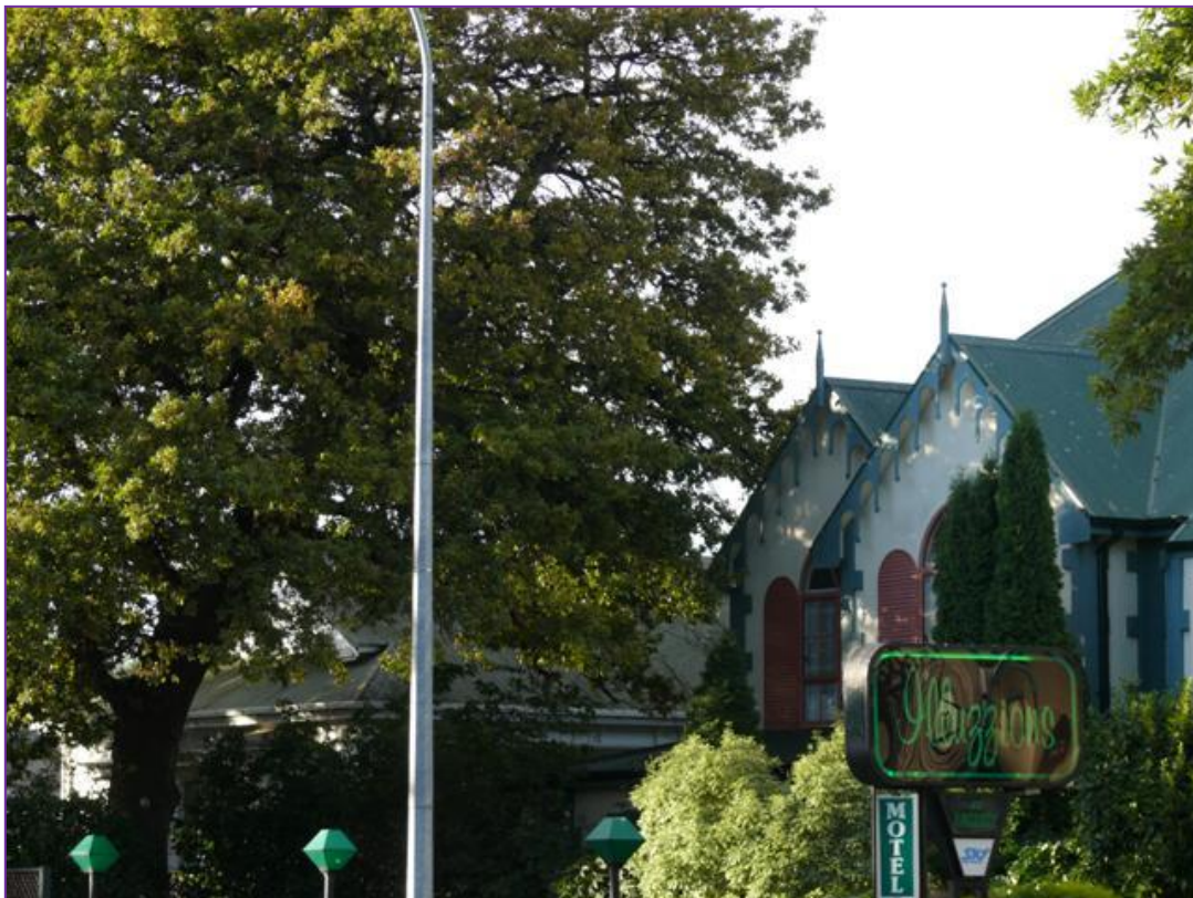
Figure 3. The overhanging branches could be reduced to give more clearance from the windows.
