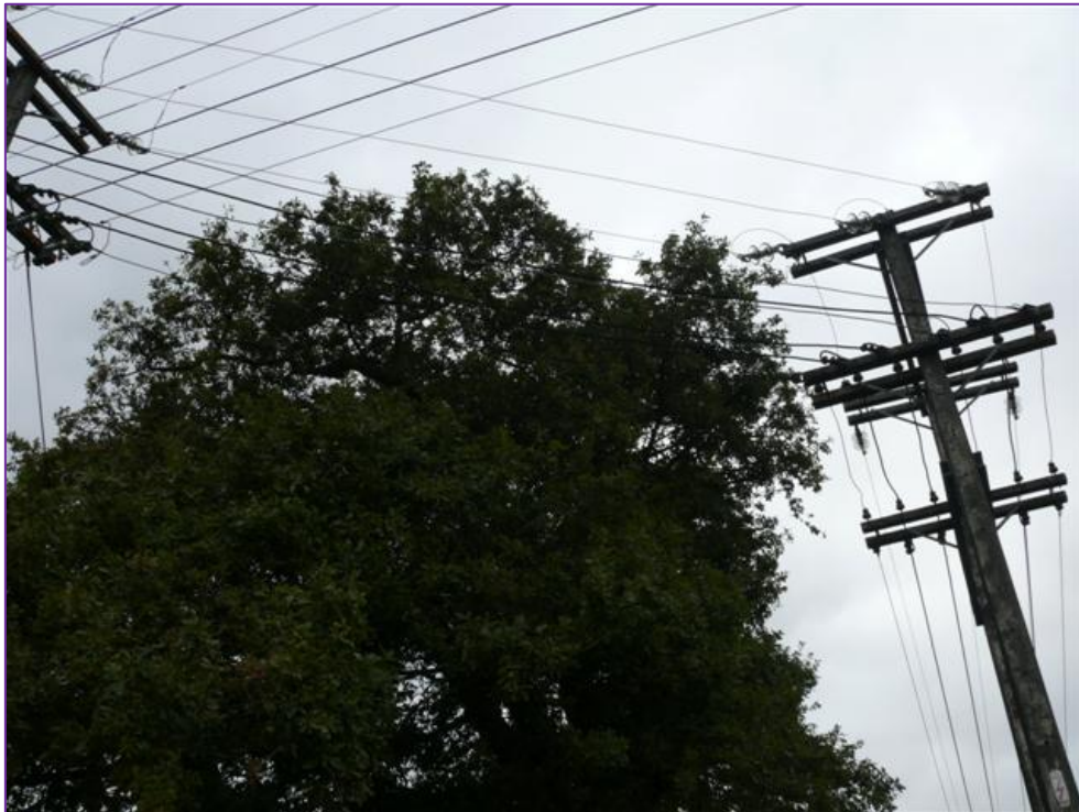
Figure 5. The challenge: to reduce the impact of the overhead lines outside the property.
