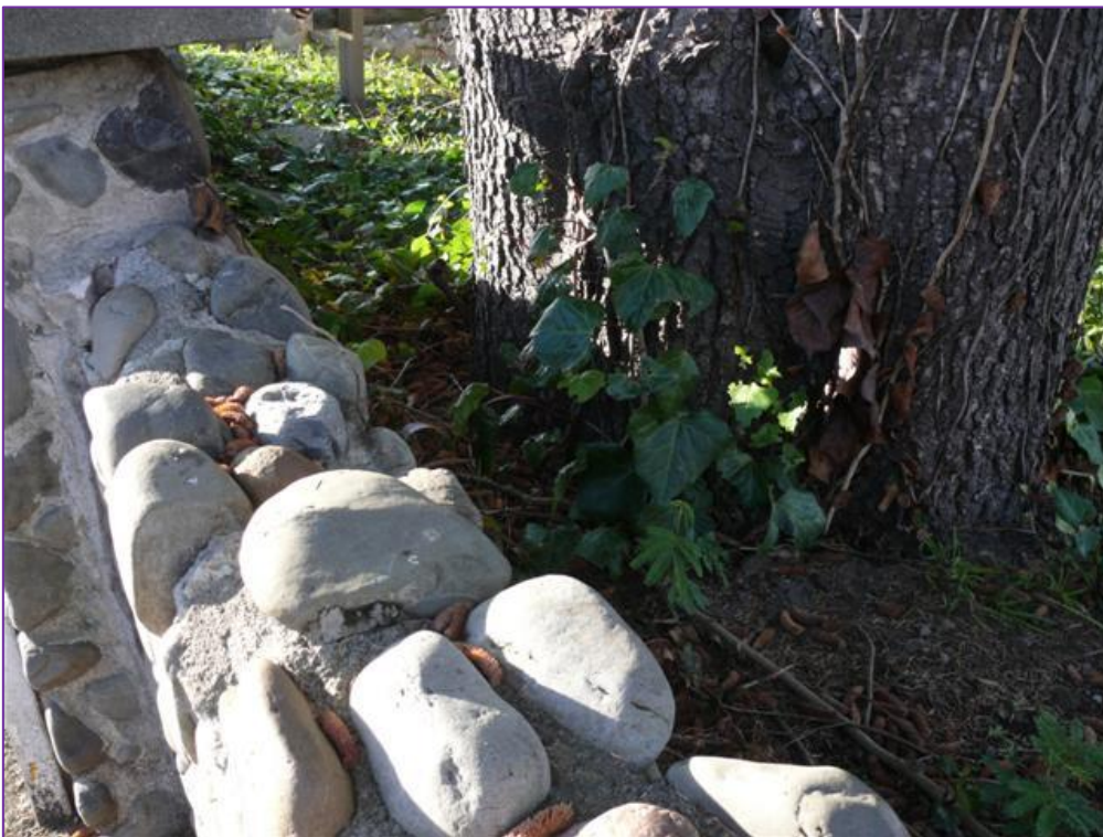
Figure 2. Detail of wall
