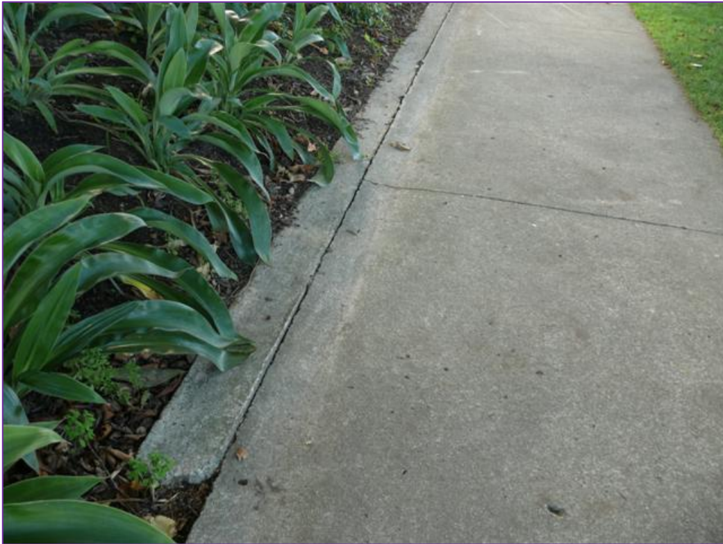
Figure 1, the footpath is intact.
