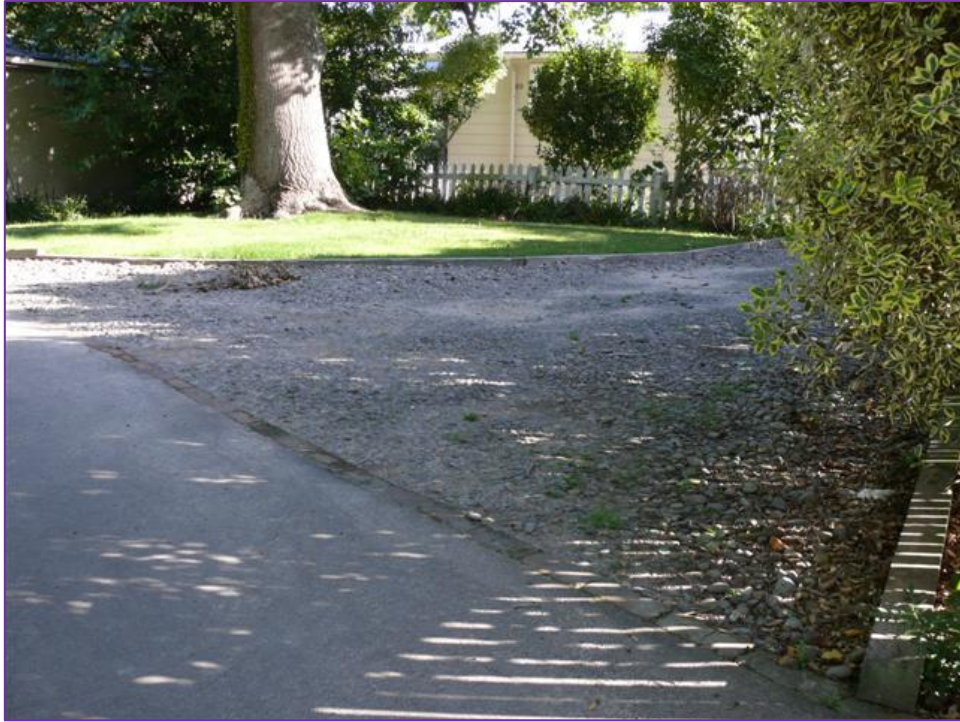
Figure 3. permeable standing is good for root development and water percolation.
